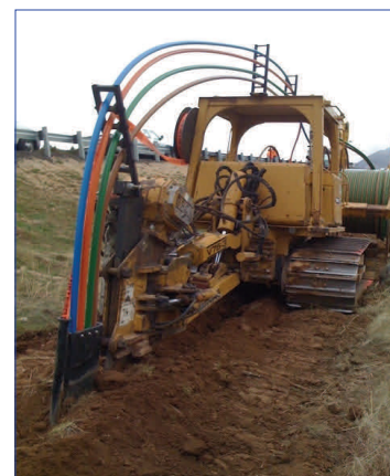
Conduit being installed along I-80 in Utah.
